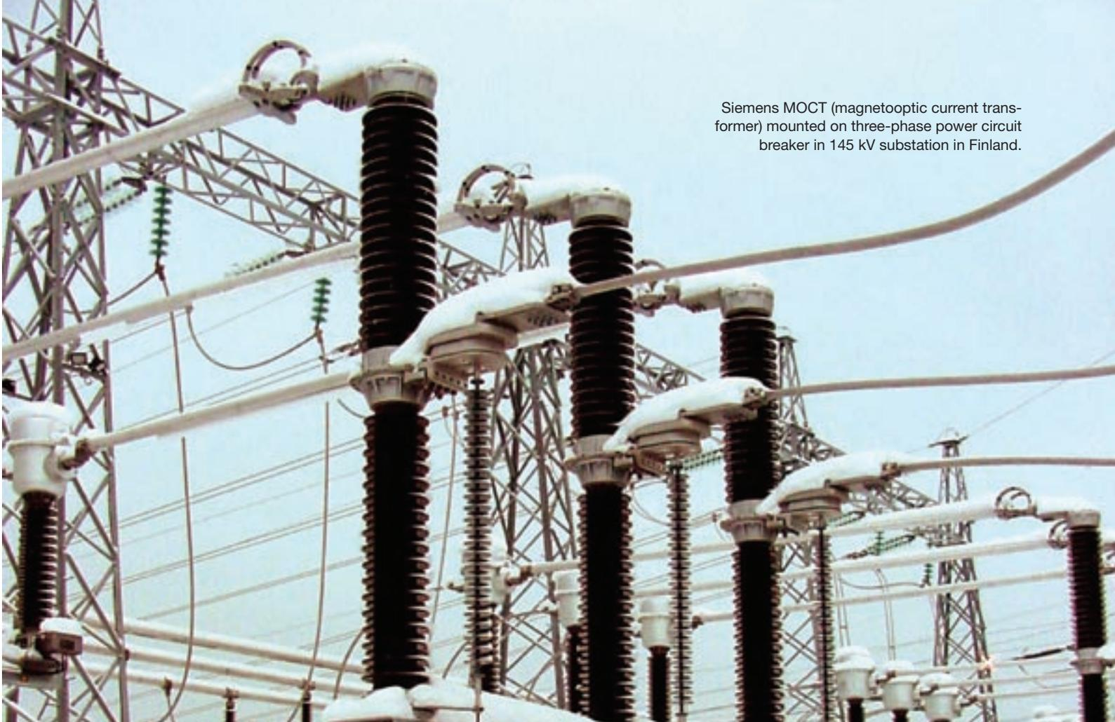
Siemens MOCT (magneto-optic current transformer) mounted on three-phase power circuit breaker in 145 kV substation in Finland.
