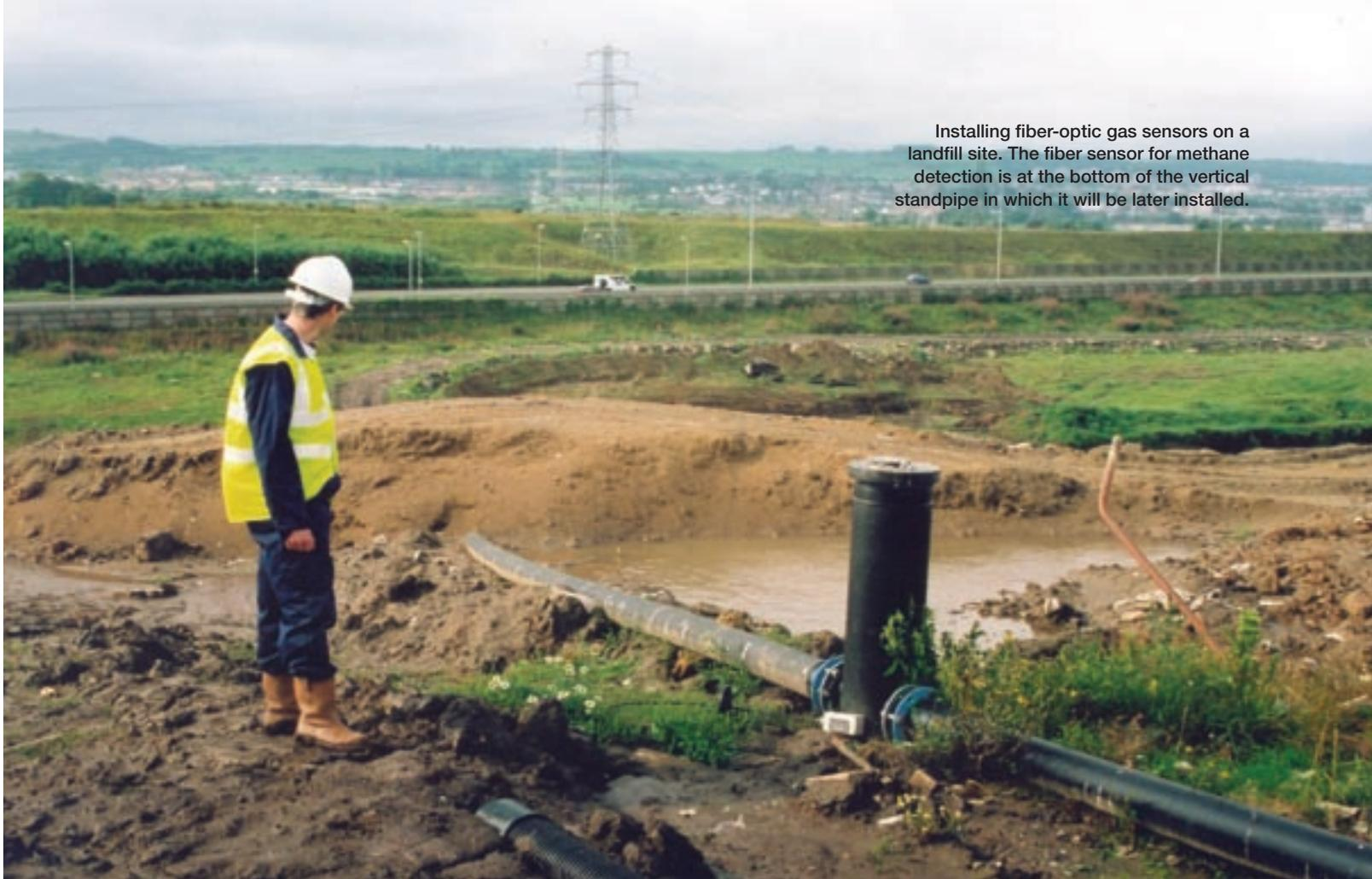
Installing fiber-optic gas sensors on a landfill site. The fiber sensor for methane detection is at the bottom of the vertical standpipe in which it will be later installed.
