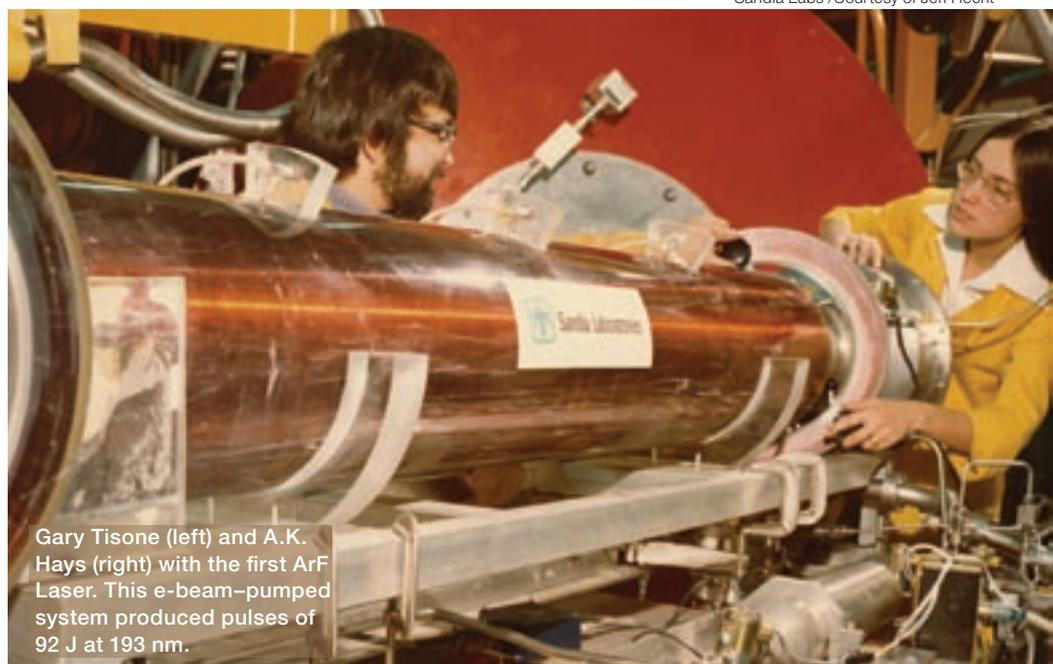
Gary Tisone (left) and A.K. Hays (right) with the first ArF Laser. This e-beam-pumped system produced pulses of 92 J at 193 nm.
